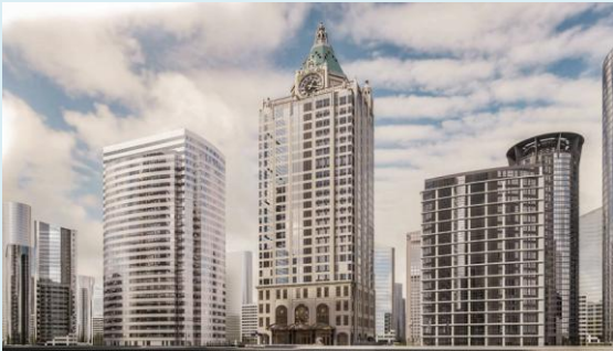
Project name: Kronos office building Country: Thailand Catchment area: 1,779.84 sqm
