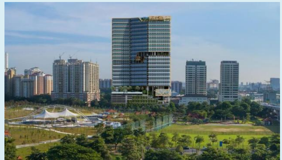
Project name: Parc 3 Country: Malaysia Catchment area: 1,690 sqm
