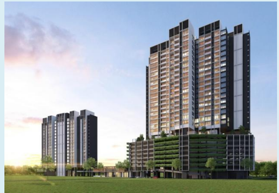
Project name: Pavilion Embassy Lot 5 Country: Malaysia Catchment area: 7,500 sqm
