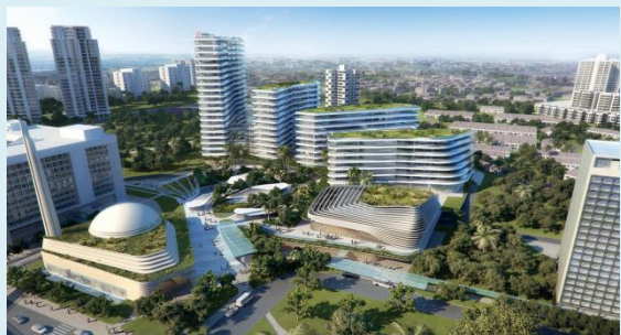
Project name: TNB Balai Islam Bangsar (Phase 1) Catchment area: 3,980 sqm
