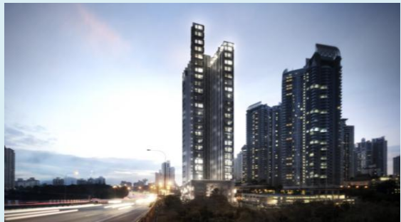
Project name: TWY Mont Kiara Catchment area: 1,660 sqm
