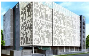
Global Switch Data Centre
