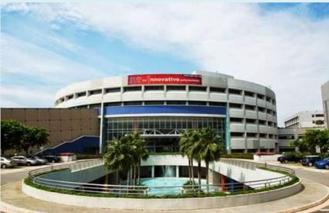
Project title: Nanyang Polytechnic Roof area: 13,500 sqm
