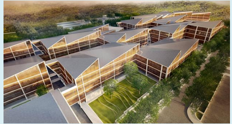
Project title: Raffles American School Roof area: 28,900 sqm
