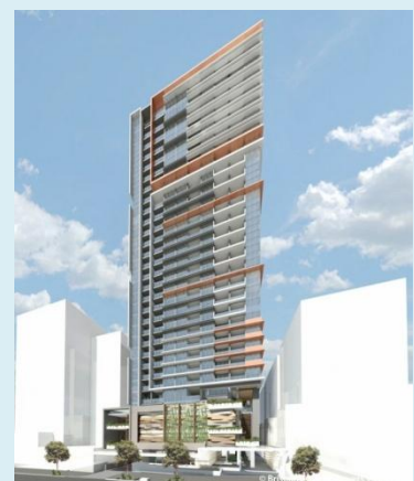
Project name: Brisbane Casino Tower Catchment area: 2,955 sqm
