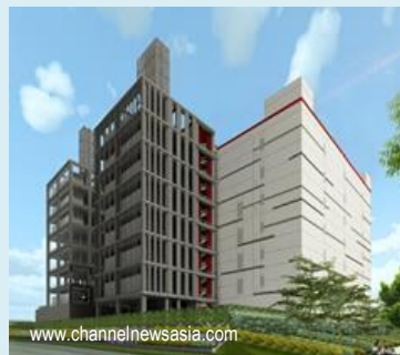
Project name: Singtel Data Centre Catchment area: 5,400 sqm
